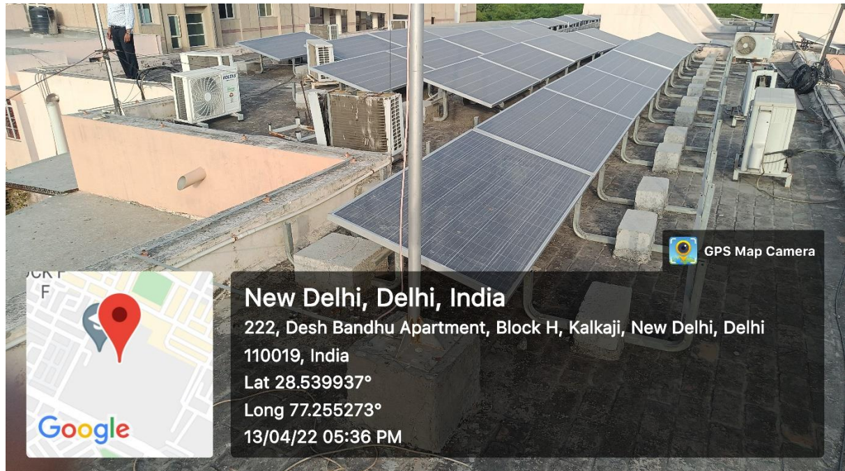
Figure 2. Library building roof with solar panels for green energy.
