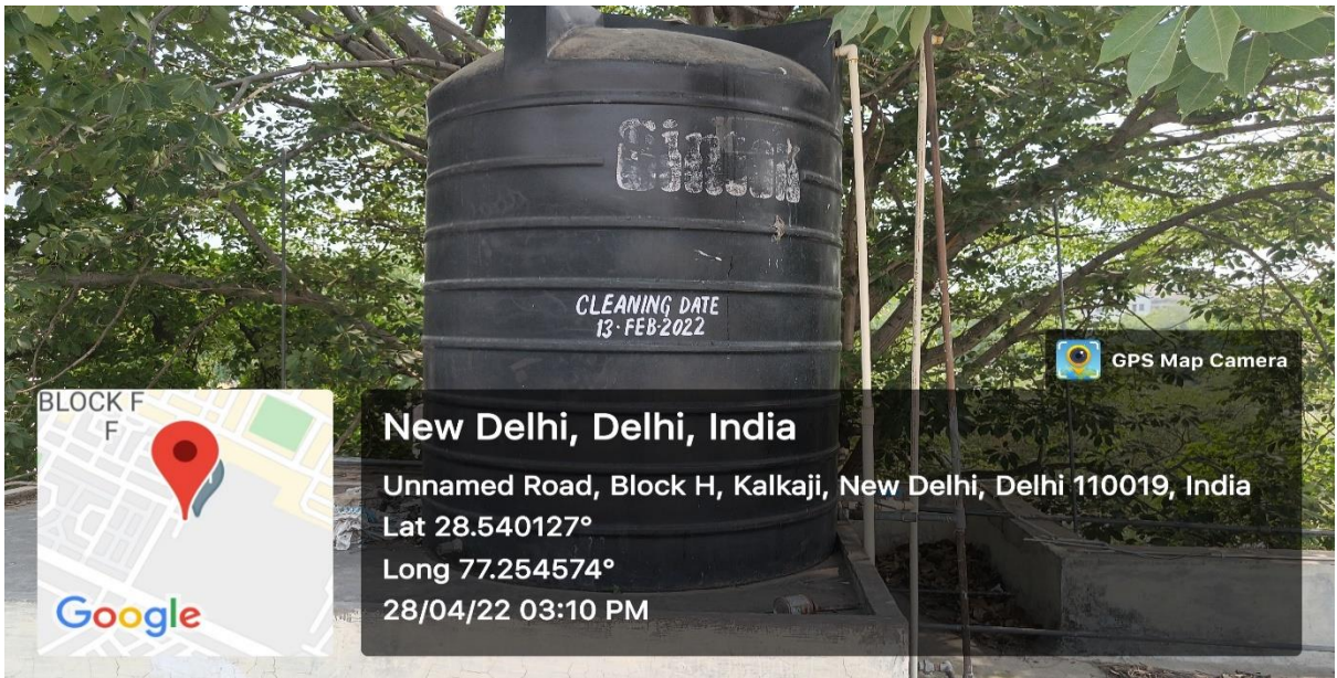
Figure.7 Water tank on the roof of the administrative block along with the latest cleaning date
