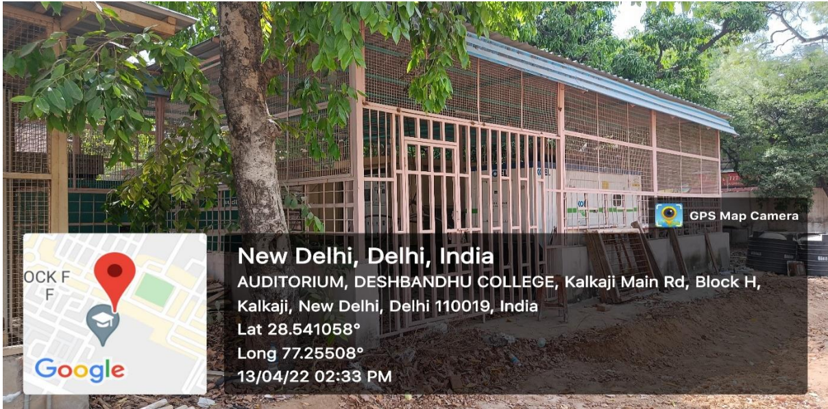
Figure.6 Modern Generator set for efficient use of electricity resources in the campus
