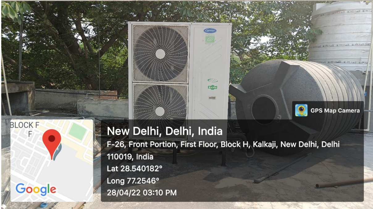
Figure.6 LED lights and central air conditioners for efficient use of electricity in the campus
