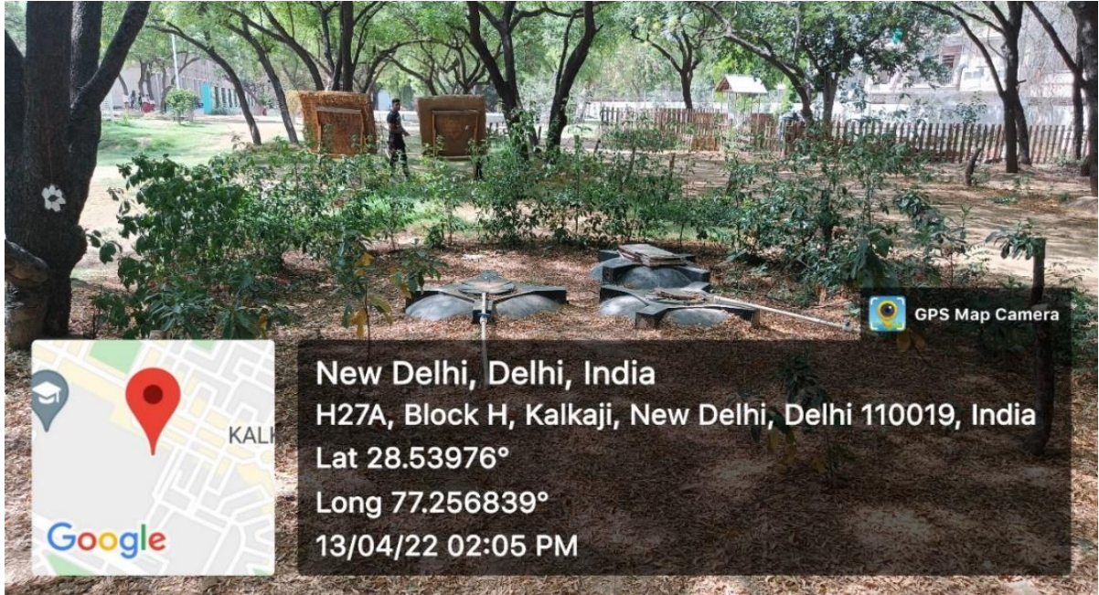
Figure.5 Waste water storage tank used for watering to the plants
