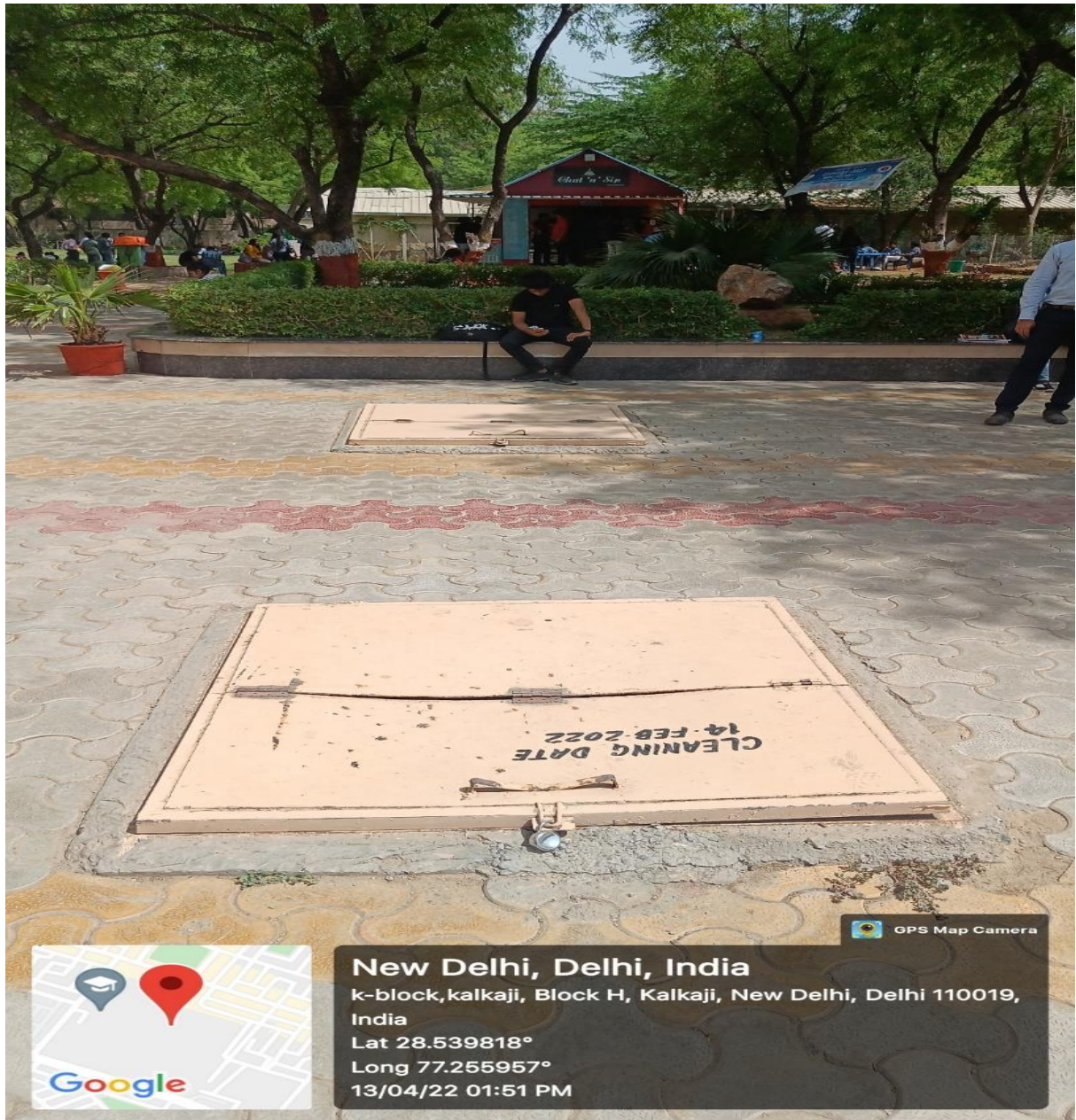
Figure 3. Water storage tank.
