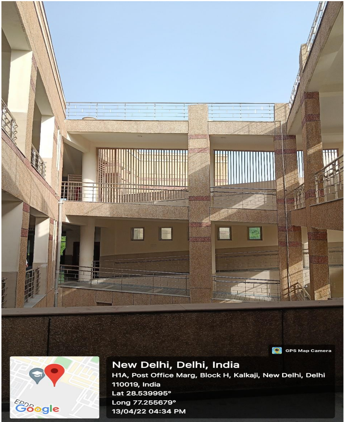
Figure.8 Wide and spacious staircase in the new block for proper ventilation and natural light in the entire building
