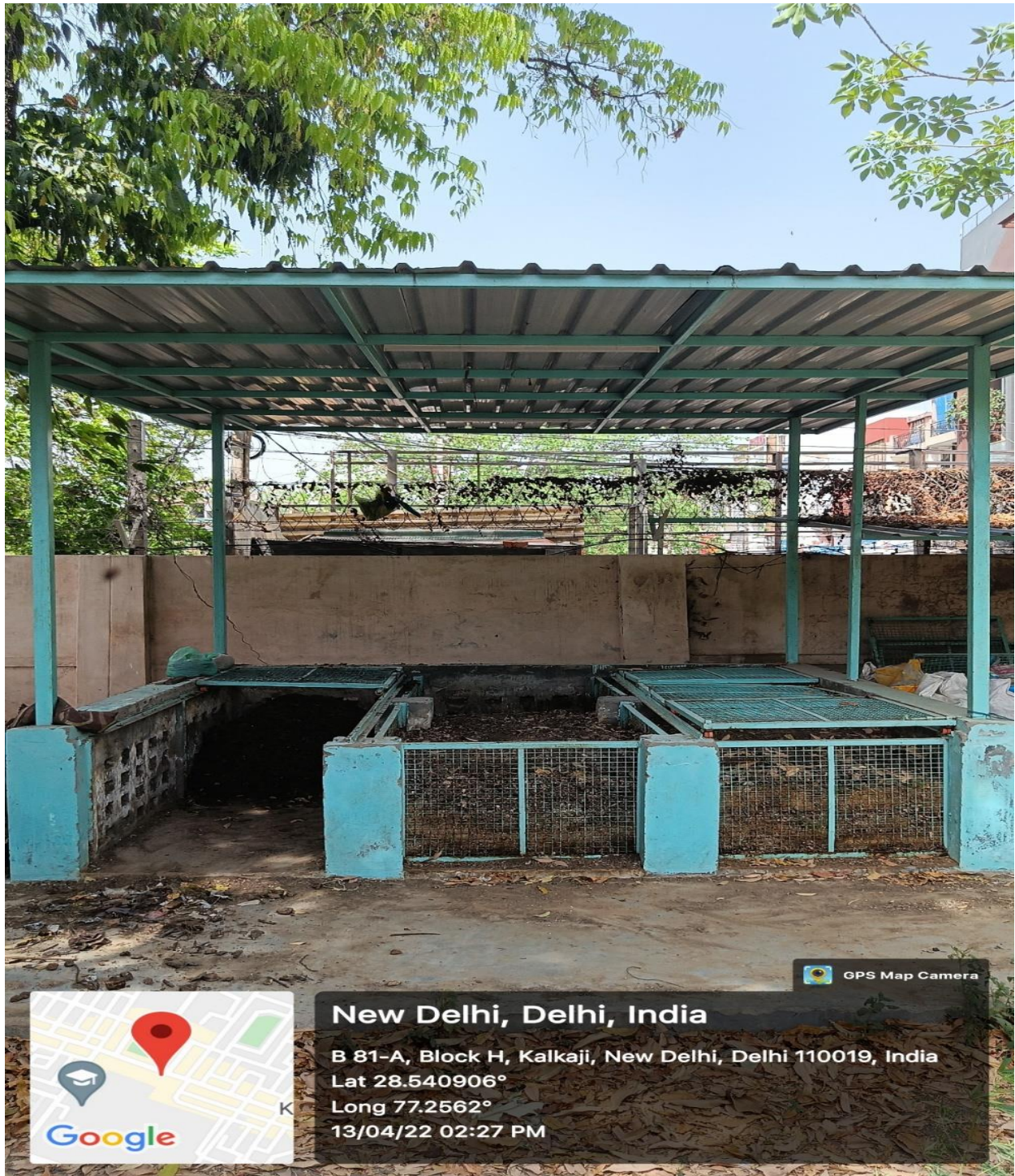
Figure 3. Composting unit for the biodegradable waste treatment
